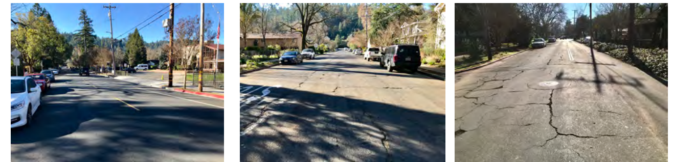
Berry Street (left), Cedar Street (middle), Washington Street (right)
