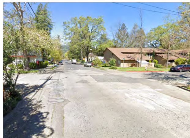
There are no crosswalks at the Berry Street and Myrtle Street intersection.
