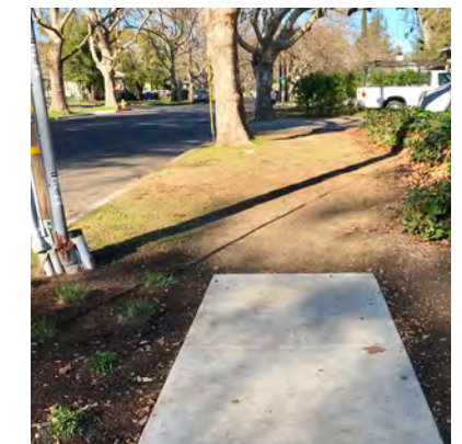
Sidewalk ends on Cedar Street
