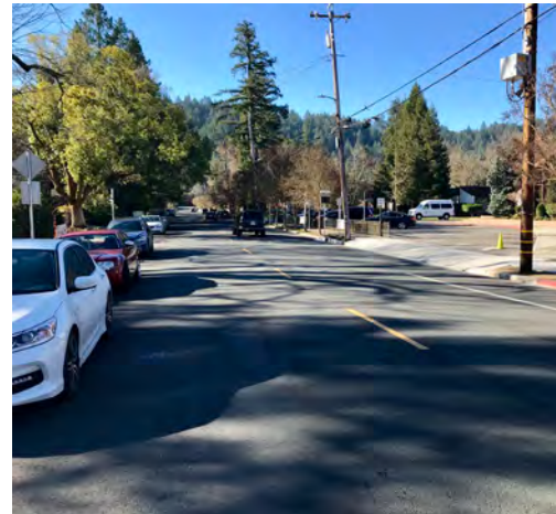
There is no midblock crosswalk that leads to the front of the school on Berry Street.
