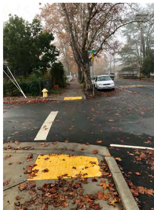
There is no crosswalk at Miriam Avenue and Lake Street.
