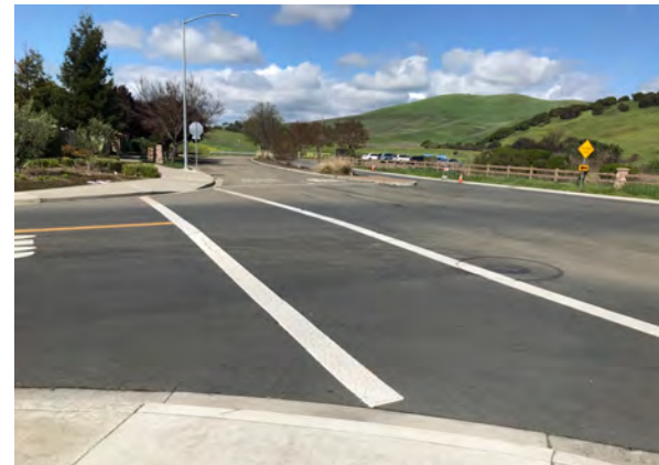
The Donaldson Way East and Newell Drive intersection, looking north.
