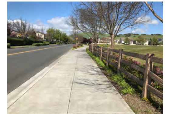
Above: Without signage or stencils, the Donaldson Way East Class I facility appears to be a pedestrian-only sidewalk.
