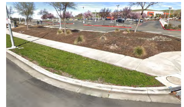
Bicyclists must share the northbound sidewalk on Newell Drive in front of the high school with pedestrians to travel to the nearest crosswalks to the Class I shared-use path on the other side of the street. The sidewalk is too narrow for shared pedestrian and bicyclist use.
