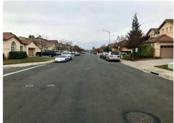
Chicanes can help reduce speeding on long, wide, straight roads such as Hummingbird Way (photographed above).
