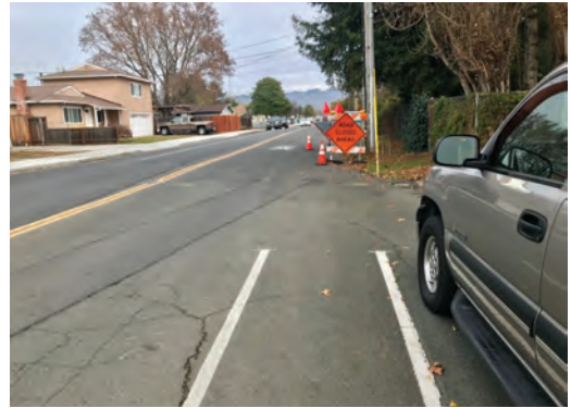
The eastbound Class II bike lane on Donaldson Way West suddenly turns into a Class III bike boulevard when the roadway narrows with no prior warning to motorists or bicyclists.
