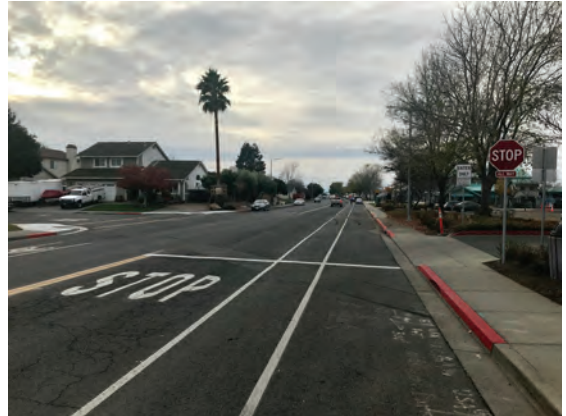
Low pedestrian visibility and vehicles failing to stop at stop signs are the major barriers at the Benton Way and Chaucer Lane intersection.
