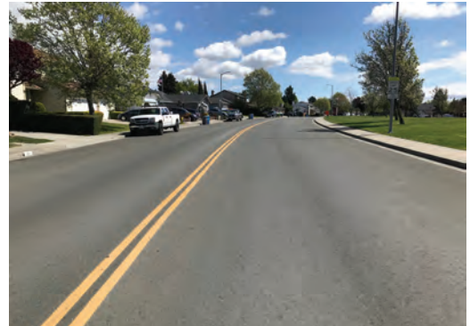
Donaldson Way, facing south. Adding Class II bike lanes and traffic-calming features would help reduce speeding by narrowing the roadway.
