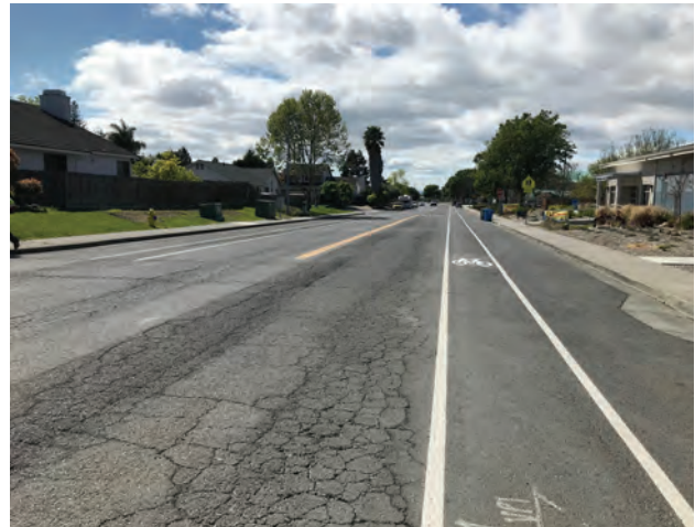
Students may be riding on the sidewalk instead of the Class II bike lanes on Benton Way due to high vehicle speeds and volumes and frequency of cars pulling up to the curb in the school area. Note: bike lane stencils were added to the bike lanes after the ACMS Walk Audit.
