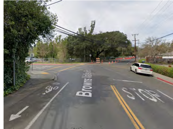
The Browns Valley Road and Buhman intersection (construction on Browns Valley Road has since been completed).
