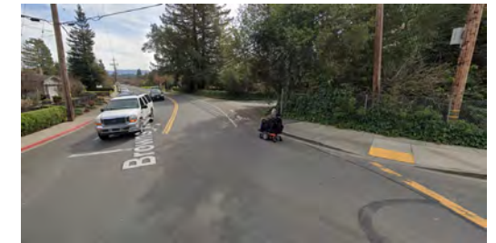
One of the sidewalk gaps on Browns Valley Road is immediately east of the Buhman intersection in front of the school.
