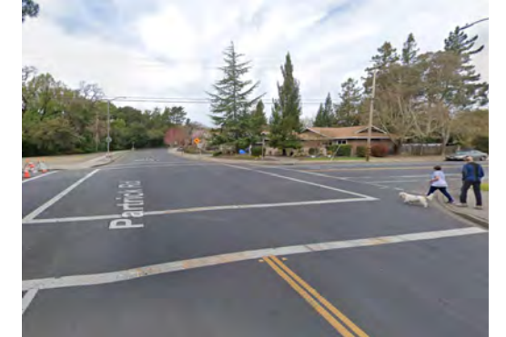
The existing crosswalks at the Browns Valley Road and Partrick Road (west) intersection are painted a low-visibility pattern.
