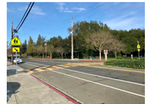
Rectangular Rapid Flashing Beacons were installed at the Buhman Avenue midblock crosswalk after the Walk Audit.
