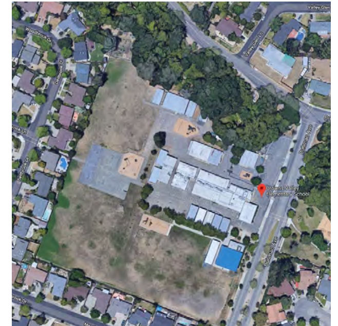
Browns Valley Elementary School's primary entrance is on Buhman Avenue to the east.
