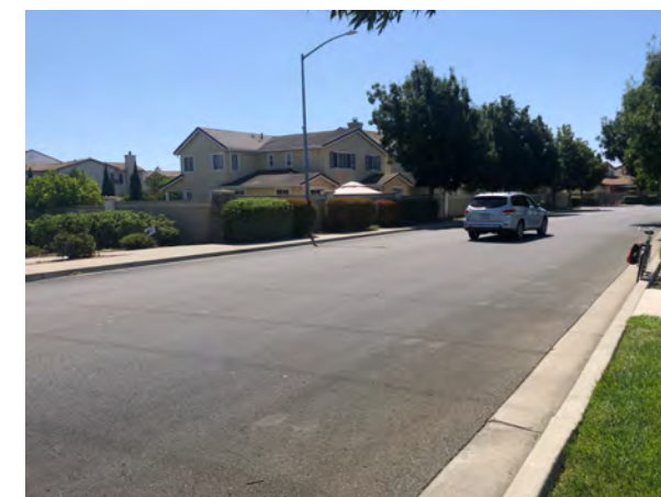
Existing conditions at the north shared-use path and Shenandoah Drive.
