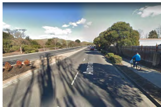
The eastbound sidewalk on American Canyon Road is too narrow for shared use.
