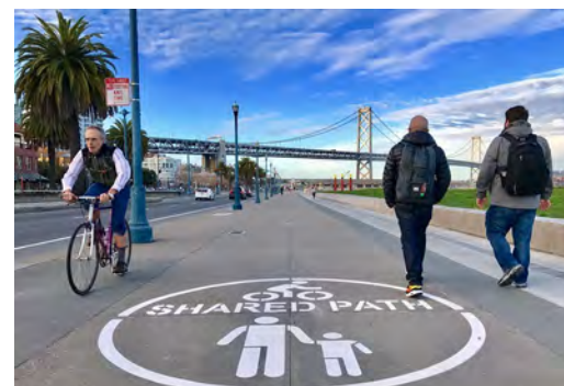
Below: Pavement stencils, as well as signage, clarify which road users can use the Class I facility (Source: SFMTA).
