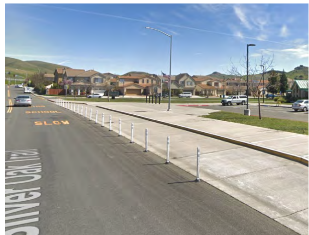
The school loading zone on Silver Oak Trail is delineated by flexiposts.
