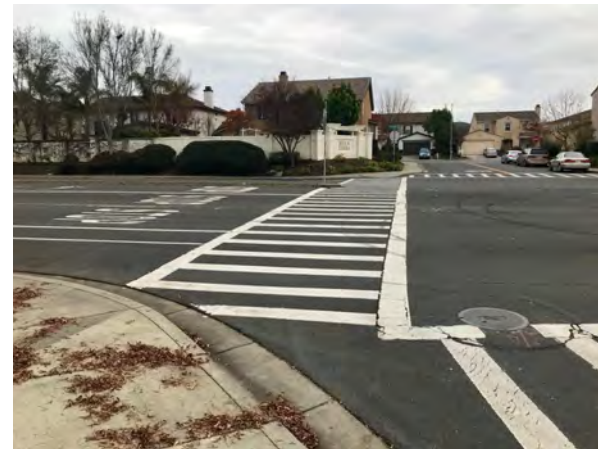
The Hummingbird Way and West American Canyon Road intersection has a long crossing distance across uncontrolled American Canyon Road traffic.
