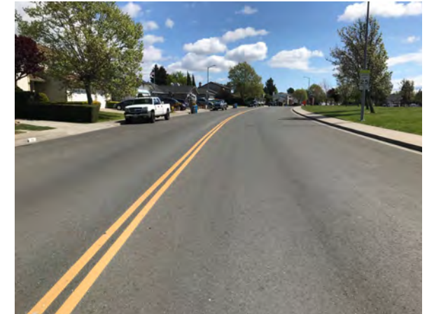
Donaldson Way, facing south. Adding Class II bike lanes and traffic-calming features would help reduce speeding by narrowing the roadway.
