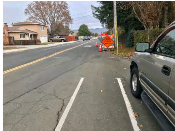
The eastbound Class II bike lane on Donaldson Way West suddenly turns into a Class III bike boulevard when the roadway narrows with no prior warning to motorists or bicyclists.
