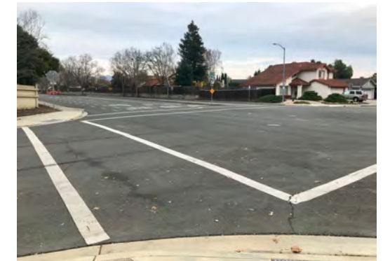
The Chaucer Lane and West American Canyon Road intersection has long crossing distances across American Canyon Road and low pedestrian visibility.
