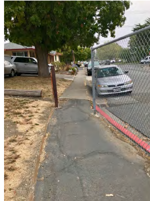
The Amarillo Drive westbound sidewalk is too narrow for the high volumes of pedestrians and bicyclists that use it to reach the school. (Note: the fencing along the sidewalk has been removed since the time of the Walk Audit).
