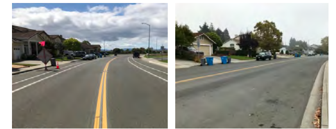
Benton Way (left) has Class II bike lanes on both sides of the road. Donaldson Way (right) has no bike facilities.
