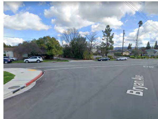
Long crossing distance at the Kilburn Avenue and Bryan Avenue intersection.
