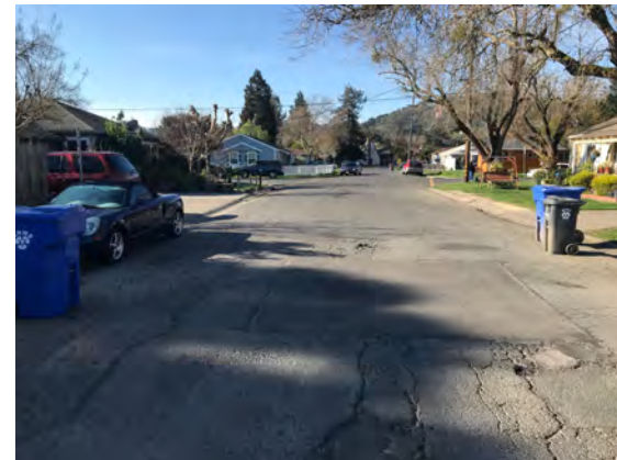
Increased streetscape lighting on Cornwall would be particularly helpful during the winter season when days are shorter.
