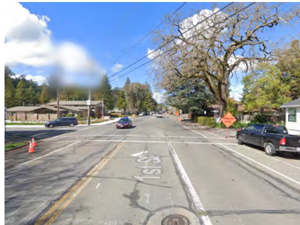
Vehicles parking adjacent to the crosswalk, shown above at 1st Street and Laurel Street intersection, reduce pedestrian visibility at an uncontrolled crosswalk.
