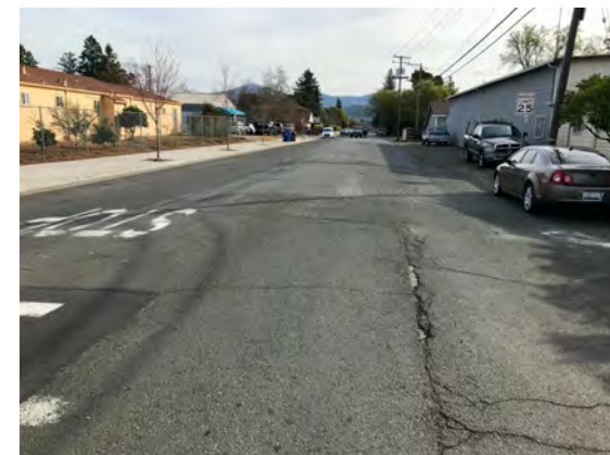
There are no bicycle facilities on Central Avenue.
