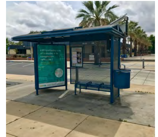
The Vine transit bus stop in front of Napa High School has a shelter and a bench.
