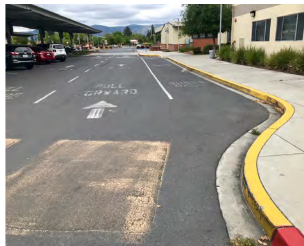
Speed cushions discourage speeding in the parking lot.
