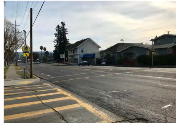
The Lincoln Avenue crosswalk has been updated to a high-visibility school-zone pattern since the time of the Walk Audit.
