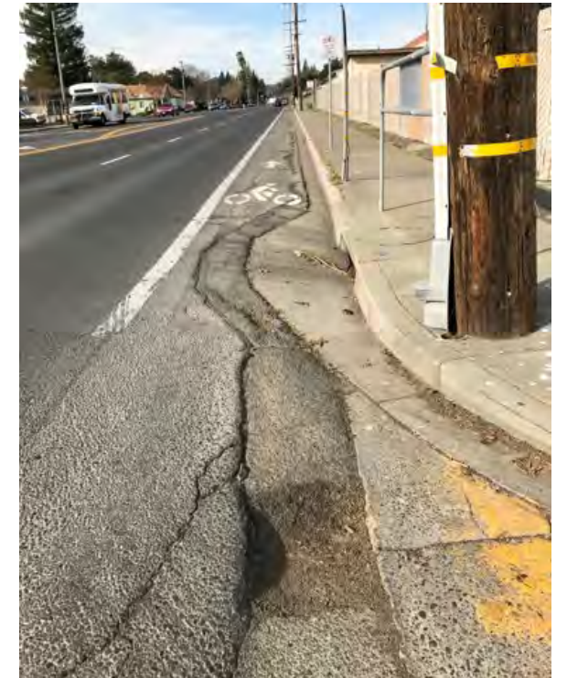
The existing Class II bike lanes on Lincoln Avenue are high-stress, which is exacerbated in areas where the bike lane is narrowed and obstructed by storm drains.
