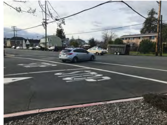
Poor sight lines cause motorists to block the crosswalk in order to see oncoming traffic.
