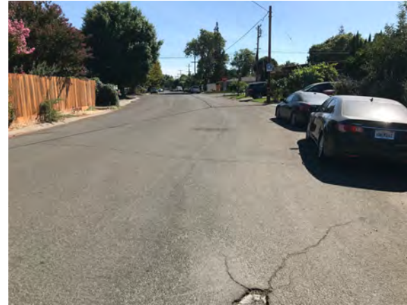
Carol Drive has no sidewalks or bicycle facilities.
