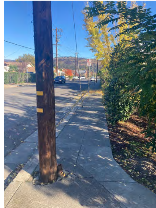
The eastbound sidewalk is obstructed by several utility and sign poles.
