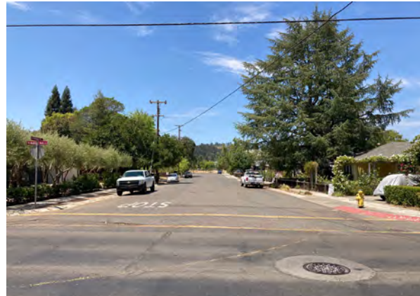
Kearney Street from Madrona Avenue to Hillview Place has more available Right of Way than the rest of the corridor, creating more opportunity for different bike facility types.
