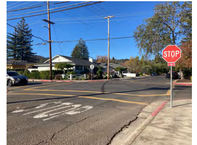
Short red curbs along Oak Avenue allow vehicles to park close to crosswalks, reducing pedestrian visibility.
