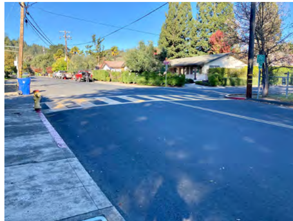
Vehicles that park adjacent to the red zone reduce visibility of crossing pedestrians to motorists.
