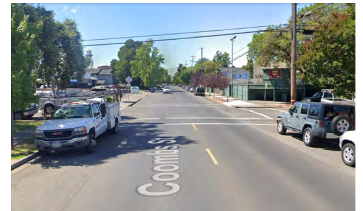
Motorists parking adjacent to crosswalks reduce pedestrian visibility.
