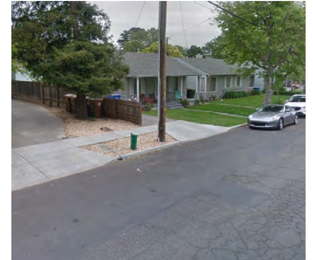
A westbound sidewalk gap on Elm Street.
