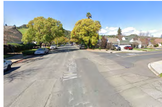
There is no crosswalk across West Imola Avenue at Kent Street.
