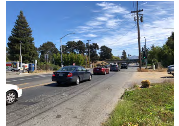
Imola Avenue has significant gaps in bicycle and pedestrian infrastructure.
