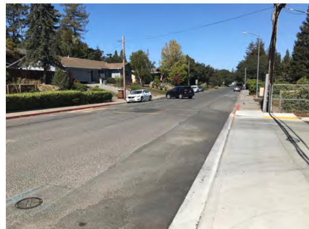
There are no bicycle facilities on Foster Road.
