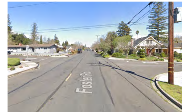
Wide curb radii at Foster and Indiana intersection allow motorists to make fast turns.
