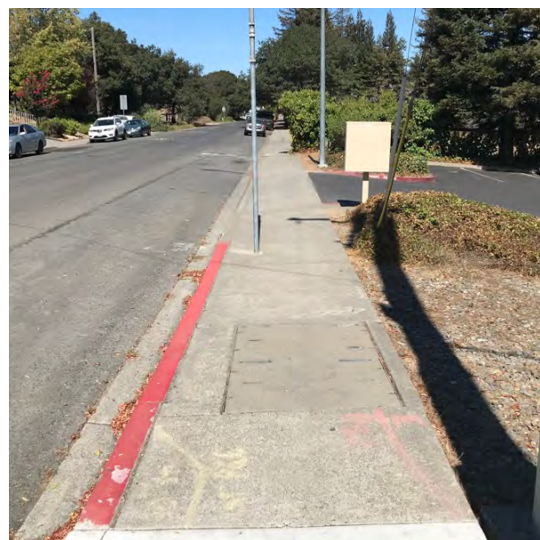
The northbound sidewalk on Foster Road.
