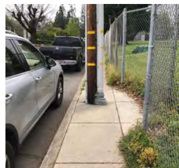
Tainter Street narrows considerably along the campus's edge – this can be a significant barrier to parents walking with strollers or people using wheelchairs.
