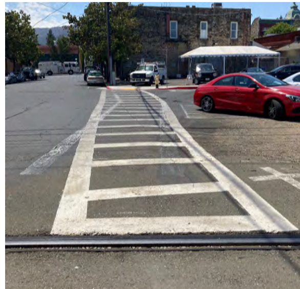
The crosswalk across Railroad Avenue at Hunt Avenue acts as an informal sidewalk to the railroad tracks. Note the obstructed visibility due to adjacent parking stalls.
