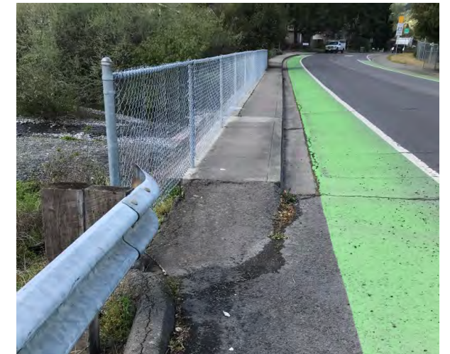
The southbound sidewalk on Valley View Street ends on the bridge over Sulphur Creek.
