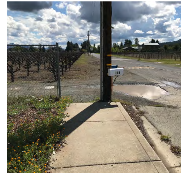
The only sidewalk on South Crane Avenue ends midblock, forcing pedestrians to walk in the dirt.
