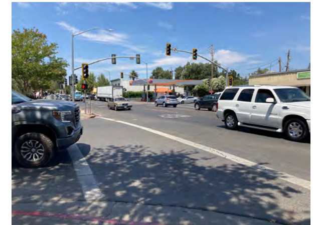
The configuration of the SR 29 and Pope Street/Mitchell Drive intersection, along with unsafe motorist right turns on red, makes pedestrian navigation of the intersection feel challenging and uncomfortable.
