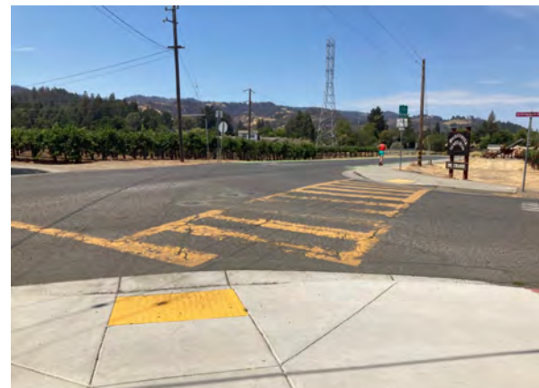
Curb extensions at Grayson and South Crane would prioritize pedestrian safety and comfort during peak school traffic hours.
