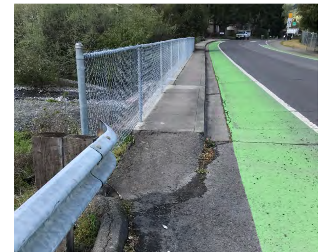
The southbound sidewalk on Valley View Street ends on the bridge over Sulphur Creek.
