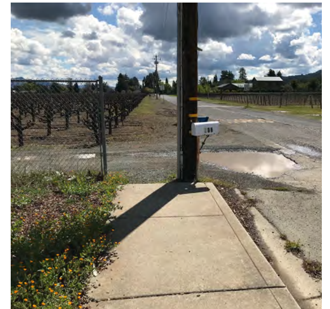
The only sidewalk on South Crane Avenue ends midblock, forcing pedestrians to walk in the dirt.
