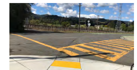
The Valley View Street and Grayson Avenue intersection is right in front of SHPS campus.
