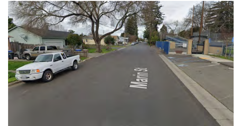
Sidewalk gaps on Marin Street.
