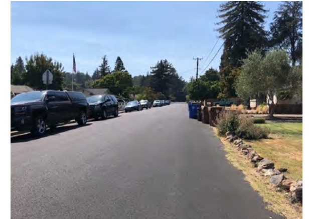
West Park Avenue sidewalk gaps can result in students walking in the street.
