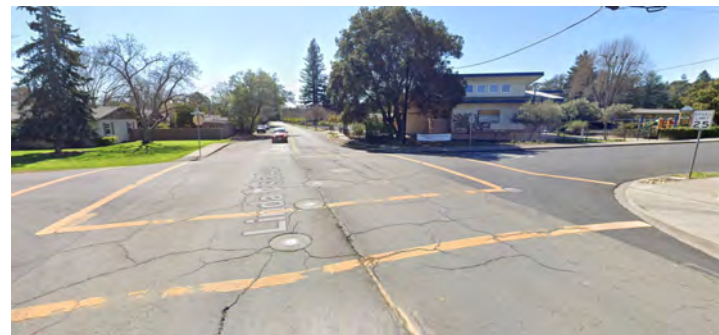
Faded, low-visibility crosswalk patterns reduce pedestrian visibility in the school zone.
