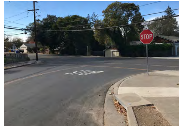
The East and Montecito intersection, facing East Ave.
