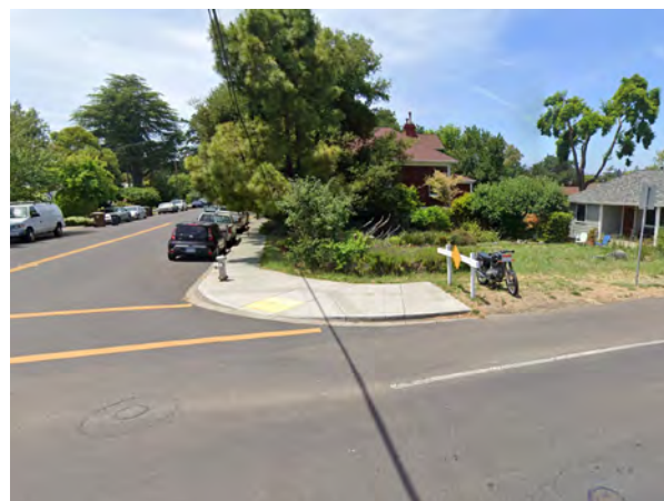
The southbound East Avenue sidewalk ends just north of the 1st Street intersection.
