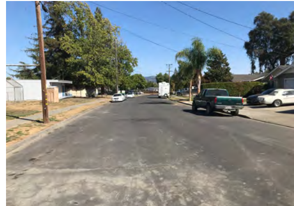
Beckworth Drive does not have bicycle facilities.
