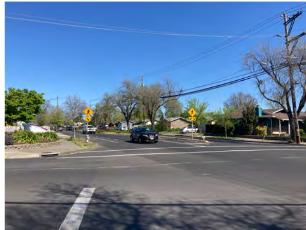
Jefferson and Rubicon intersection, facing north.
