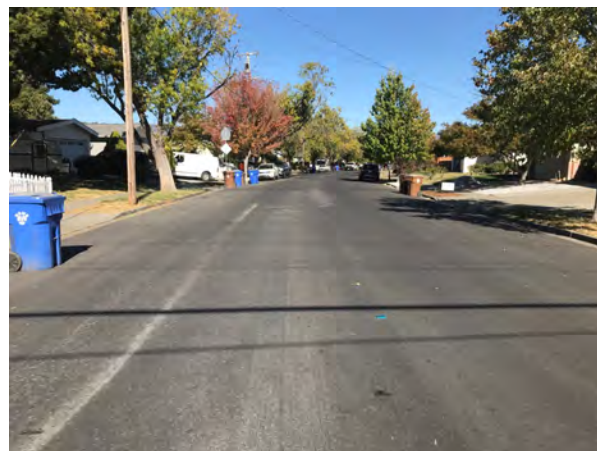
There are no bicycle facilities on El Capitan Way.
