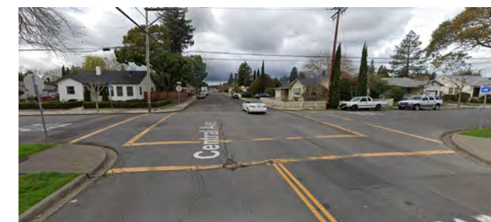
Central and Yajome intersection, facing west.
