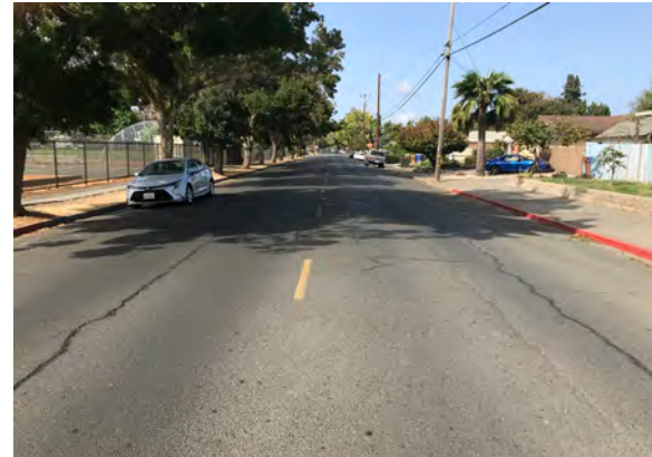
There are no bicycle facilities on Pueblo Avenue.
