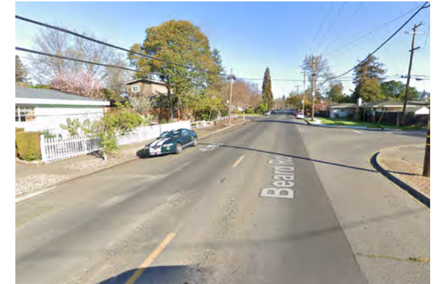
Sharrows on Beard Road indicate that bicyclists should ride next to parked cars in the door zone.
