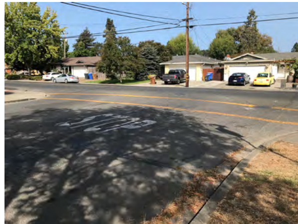
Yajome and Pueblo intersection, facing north.
