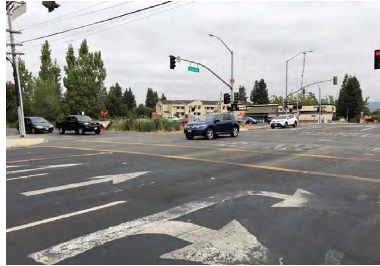
The Trower Avenue and Solano Avenue intersection.
