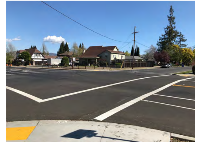
The Trower Avenue and Linda Vista Avenue intersection.
