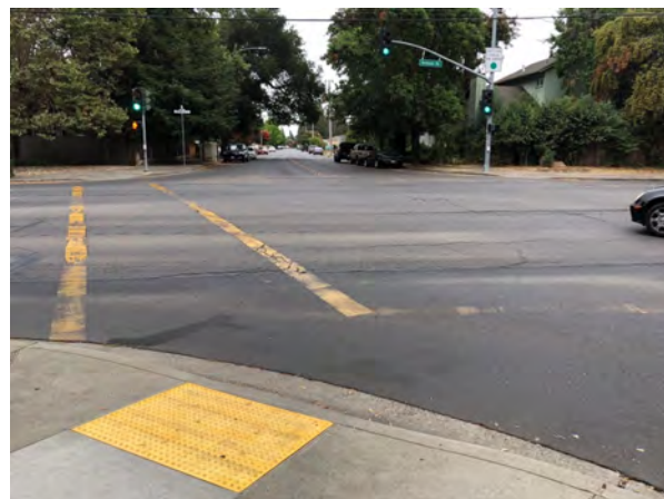
Redwood Road and Linda Vista Avenue intersection looking north.
