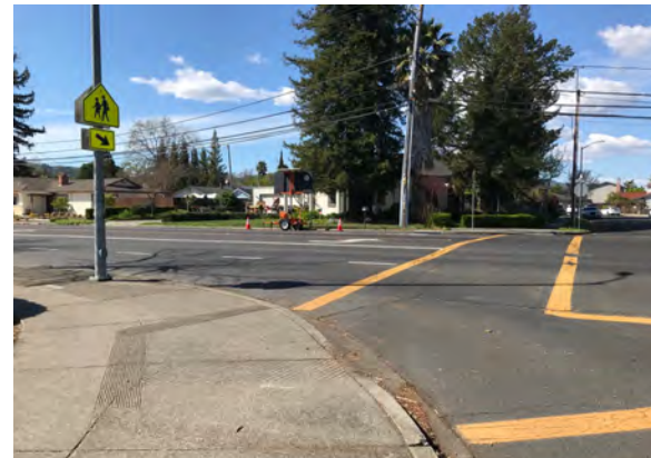
Uncontrolled traffic on Trower Avenue makes crossing the intersection at Oxford Street challenging for pedestrians.
