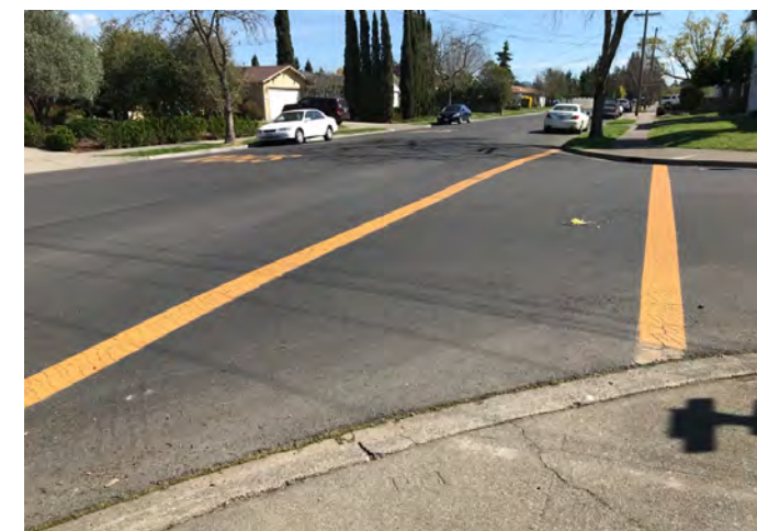
Pushed back curbs at Oxford Street and Berks Street increase crossing distance for pedestrians.
