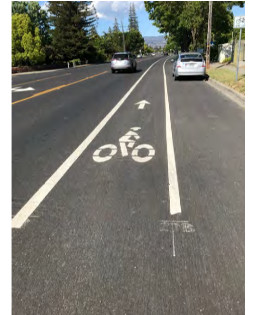
Trower Avenue currently has Class II bicycle lanes.
