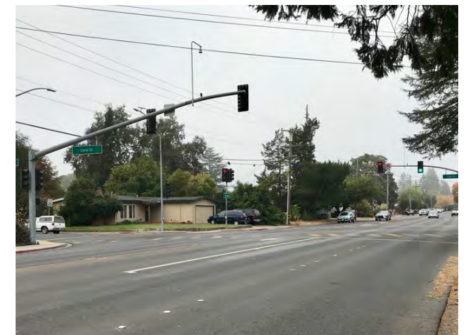
The offset intersection configuration increases pedestrian crossing distance across Redwood Road.
