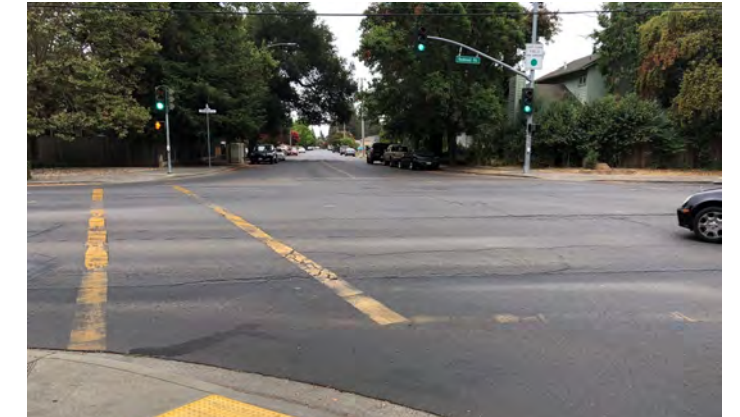
Redwood Road and Linda Vista Avenue intersection looking north.
