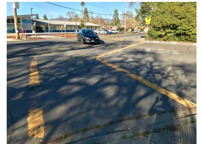
The set-back curb on Byway East extends crossing distance and facilitates fast motorist turning movements.
