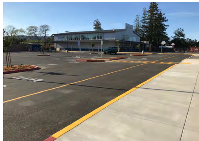
The loading zone is located in the larger, parent-use parking lot.
