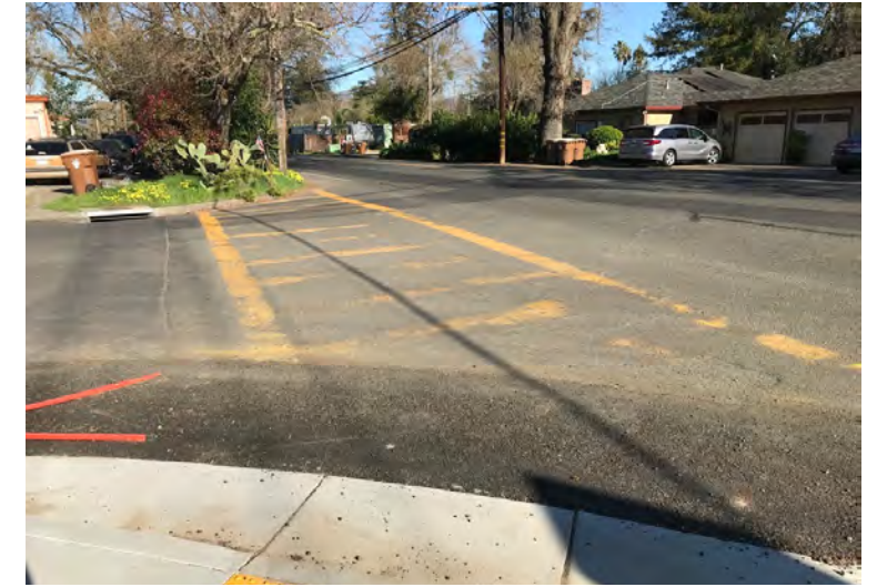
The crosswalk across Escuela Drive is extremely faded.
