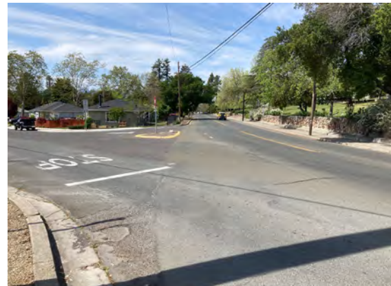
Coombsville and Linnell/Hennessy intersection, facing west.
