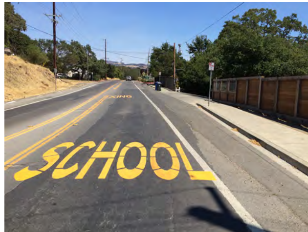
Coombsville Road approaching the school.
