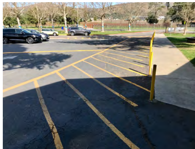
School loading zone
