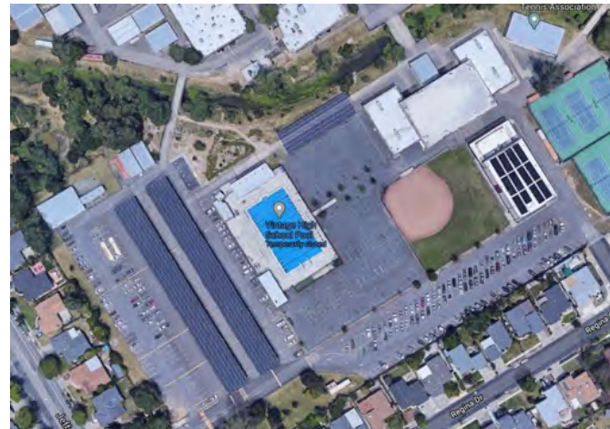
The Jefferson Street parking lot.
