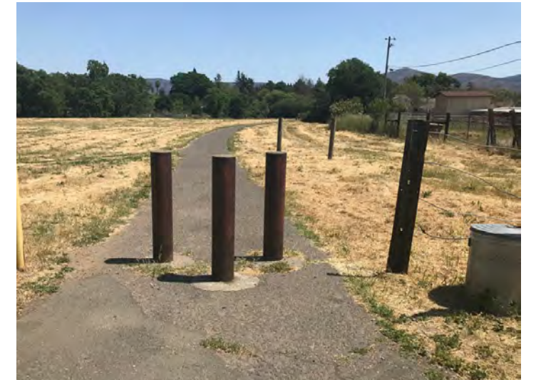
Several bollards at the entrance to the Austin Miller memorial path make entering the path on a bike challenging.
