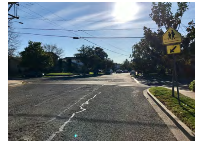
The Gordon Drive and Plass Drive crosswalks have a low-visibility crosswalk pattern.
