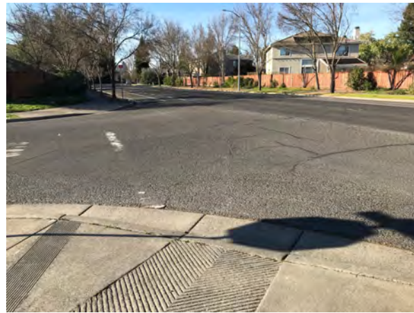
There is no crosswalk across Gordon Drive at Jefferson Street.
